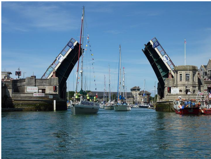
Figure 4. Town Bridge fully opened
