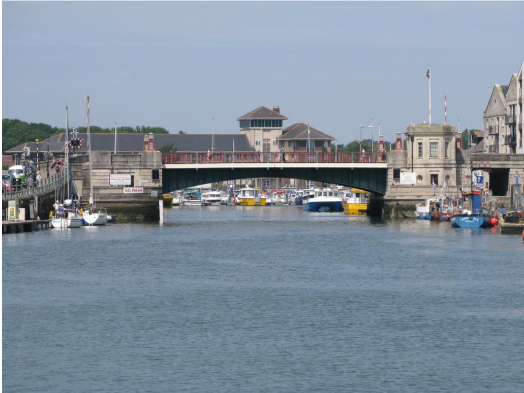
Figure 3. Town bridge closed
