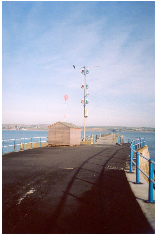
Figure 12. Movement control signal tower on South Pier end
