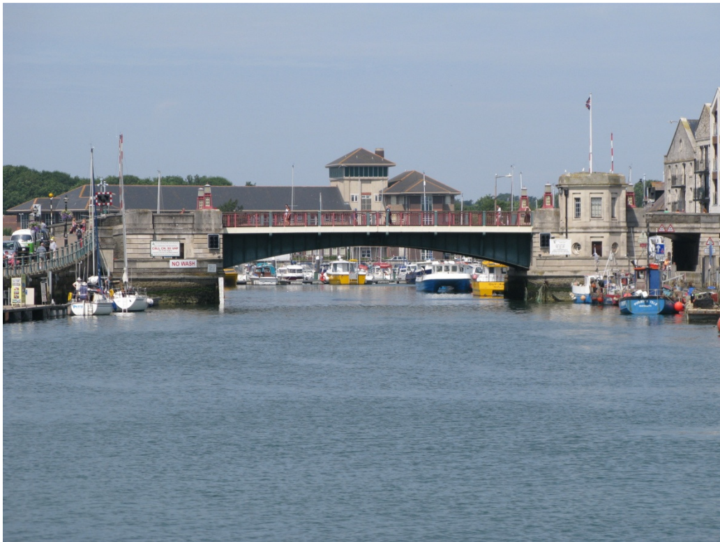
Figure 3. Town bridge closed
