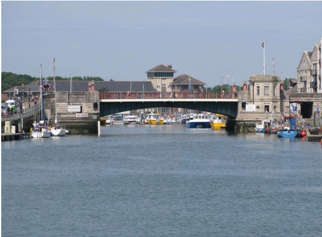
Figure 3. Town Bridge closed
