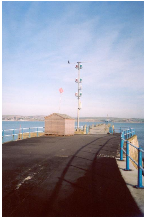
Figure 13. Movement control signal tower on South Pier end
