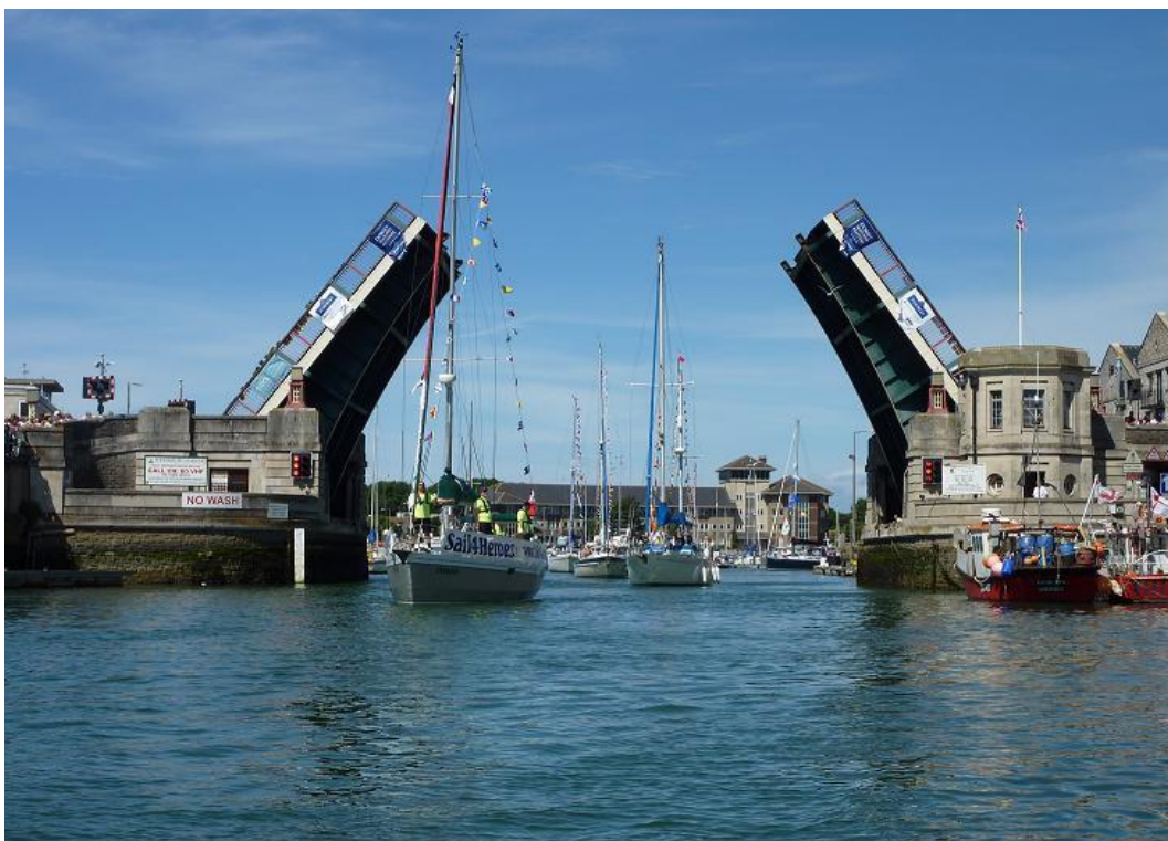
Figure 4. Town Bridge fully opened
