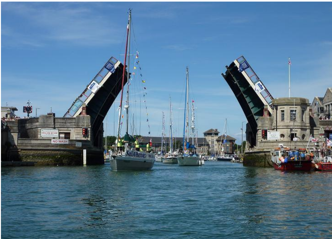
Figure 4. Town Bridge fully opened
